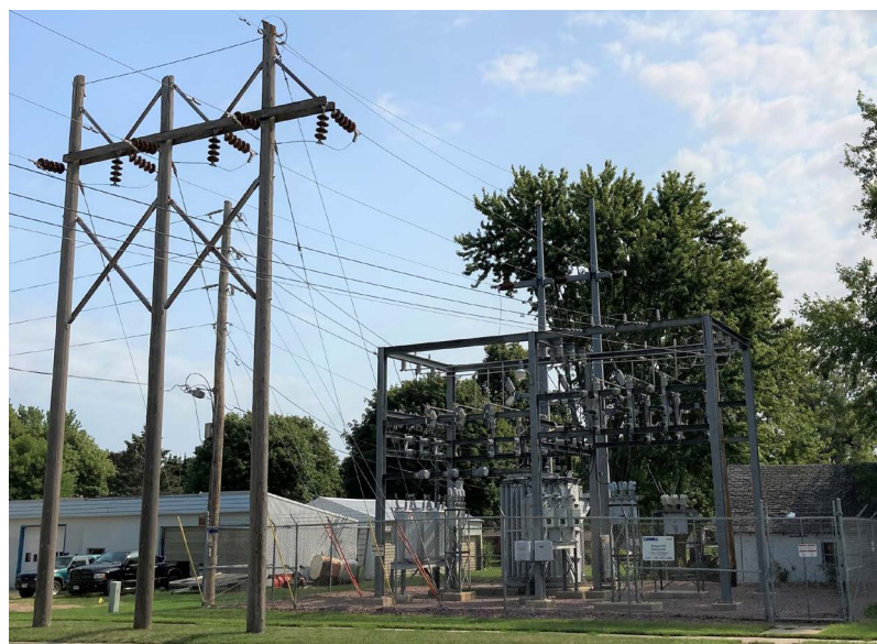
The current substation located on Hwy 4 in Trimont will be removed. A junction box will be put in its place. In addition, some of the poles near the substation will be removed.
