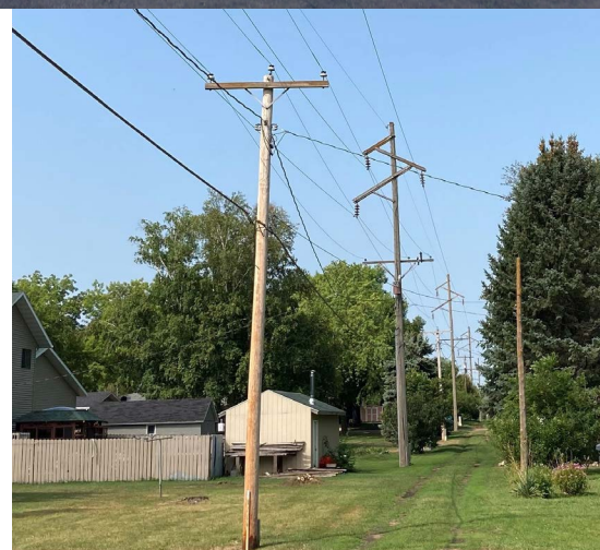
The transmission line (top line) on the west side of Hwy 4 through the alley to the current substation will be removed. The poles carrying the transmission line will stay in place. These poles also carry our distribution feed for the northwest side of Trimont. The lines on top will be removed and the poles will be shortened.
